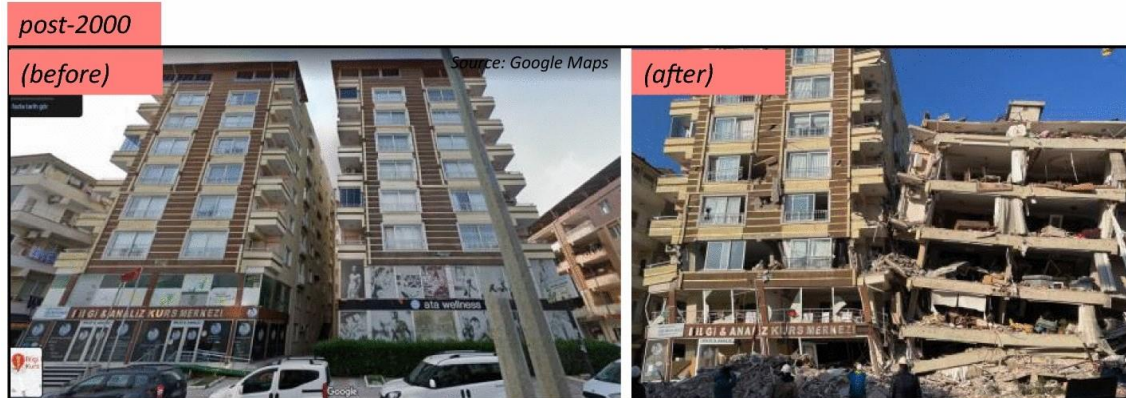
Figure 4. Collapse of Two Identical Buildings Due to Soft-Storey Mechanism in Hatay. (Vuran, E., et al. 2023)
