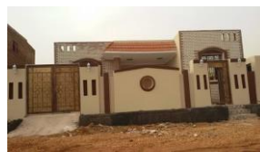
Picture 1. An external view of a detached house in Sudan
