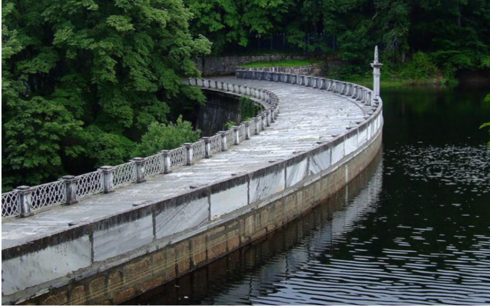
Figure 1. Sultan Mahmud Bendi with curved walls [5]
