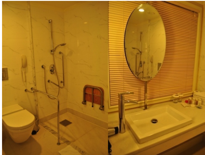
Figure VII. A well designed shower unit, but unsuitable sink height with a non-inclined mirror (Rixos Downtown, Antalya).
