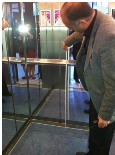
Figure IV. An elevator cabin covered with mirrors on three walls is not the right choice. The elevator walls should not be fully covered by mirrorstop revert vision disorder and disorientation. However, the elevator meets the standards in terms of measurements (Limak Artlantis Resort, Belek).
