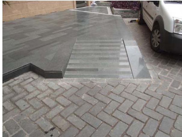
Figure II. The pavement ramp of entrance at Ramada Hotel, Antalya
