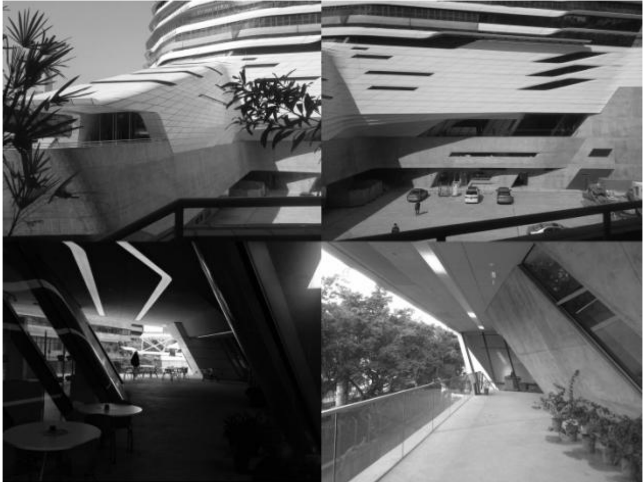
Figure 6. JCIT Strip shading devices versus strip windows (photographs: author)
