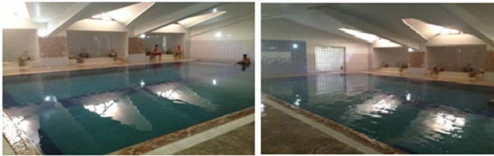
Figure 7 a, b Steam control in the units is achieved by skylights and small natural ventilation holes in the walls
