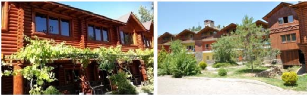
Figure 10 a, b The settlement of the accommodation units in the Kös TTFs
