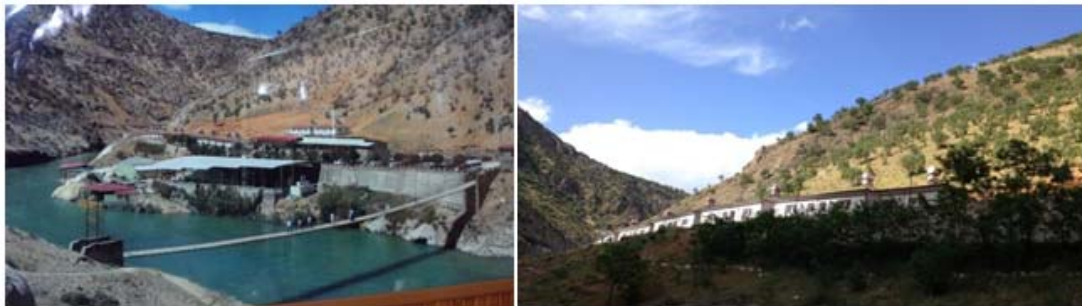
Figure 4a, b The terrain settlement of accommodation units in the Golan thermal facilities
