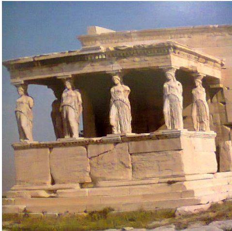
Plate 3-an ancient building with Sculptural columns as support
