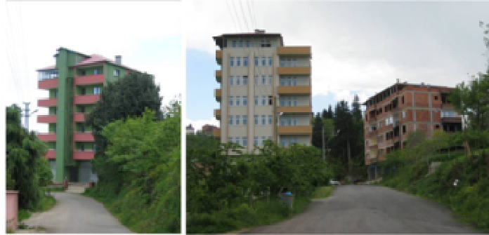
Figure 10. Settlement patterns incompatible with rural architecture (Aydın, 2010)
