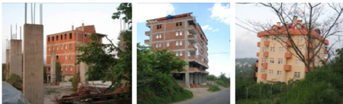
Figure 9. Reinforced concrete village houses (Aydın, 2010)
