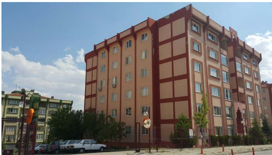
Figure 2. Facades of Selcuk Univesity TOKİ houses
