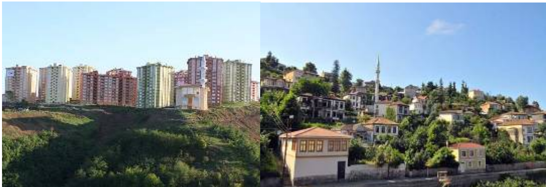
Photo 2. Location of Ortamahalle traditional houses
