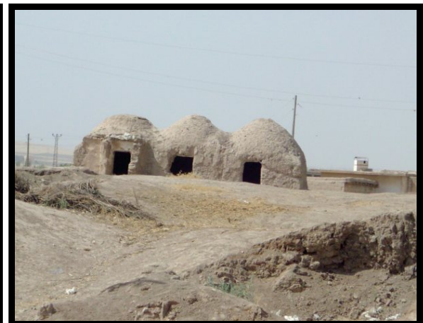
Figure 5. A view of different units
