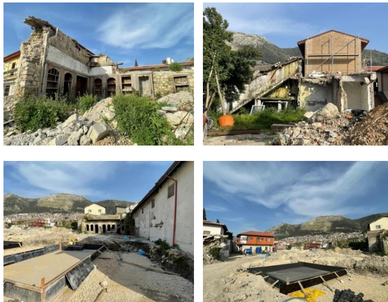
Figure 1. Post-Earthquake Destruction in Antakya (Photos by the author.)
