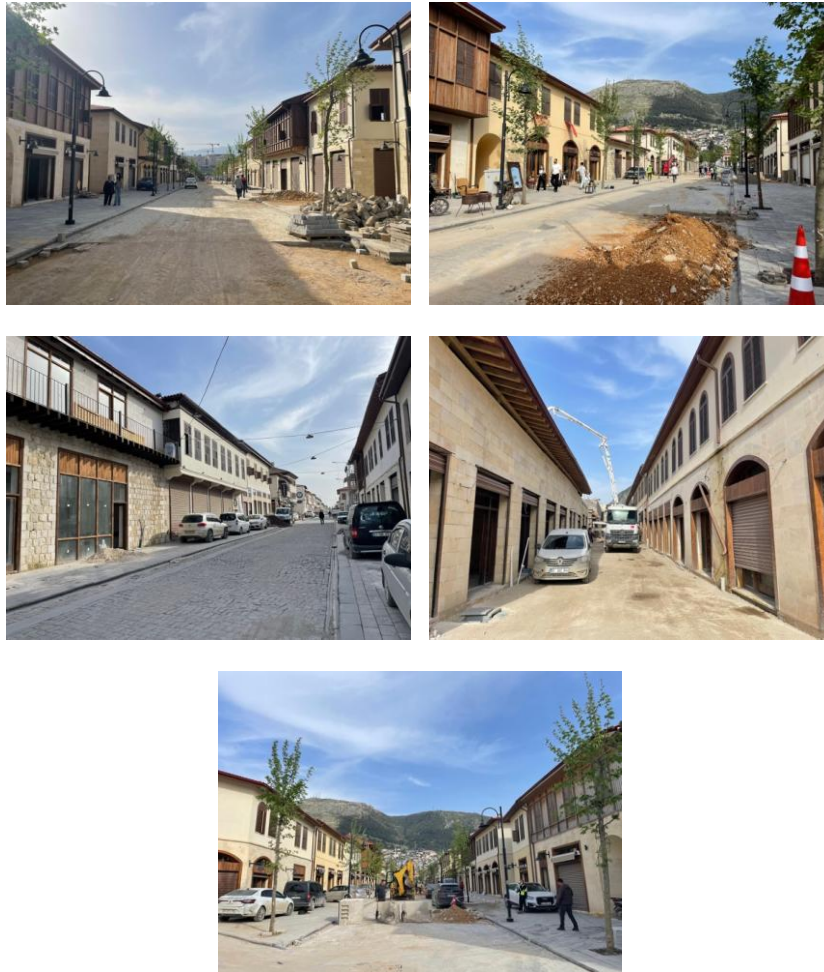
Figure 3. Post-Earthquake Street Condition in Antakya (Photos by the author.)
