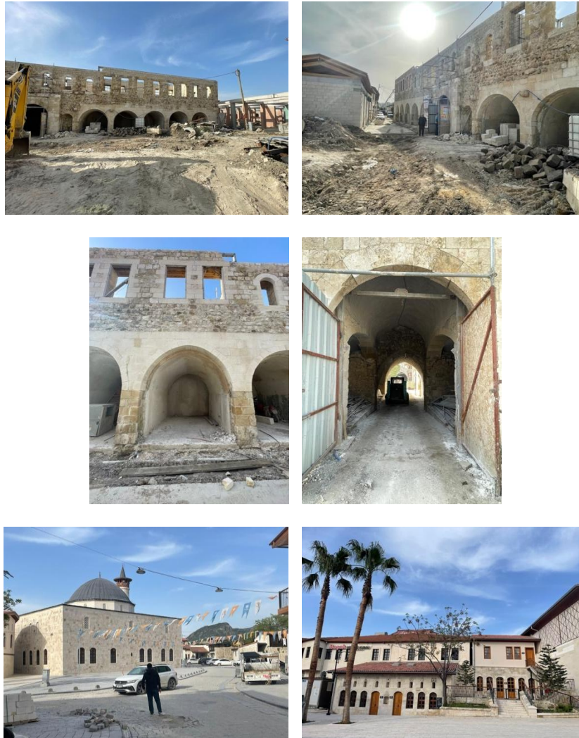
Figure 4. Restored Structure in Antakya After the Earthquake (Photos by the author.)
