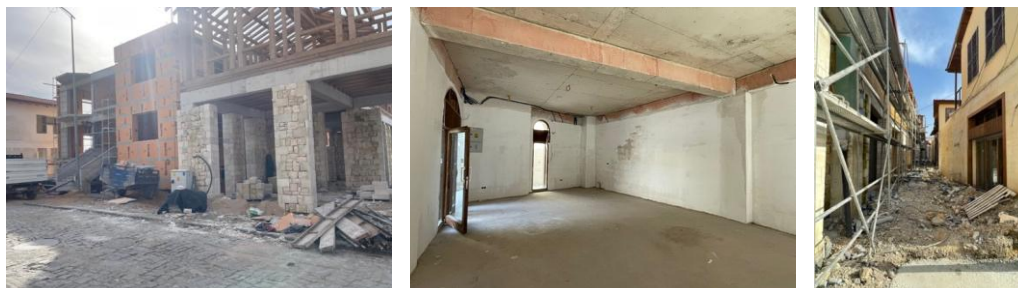
Figure 2. Post-Earthquake Construction Site in Antakya (Photos by the author.)
