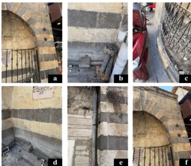
Figure 7. Chemical deterioration observed at the Köseç Ahmet Ağa Fountain
