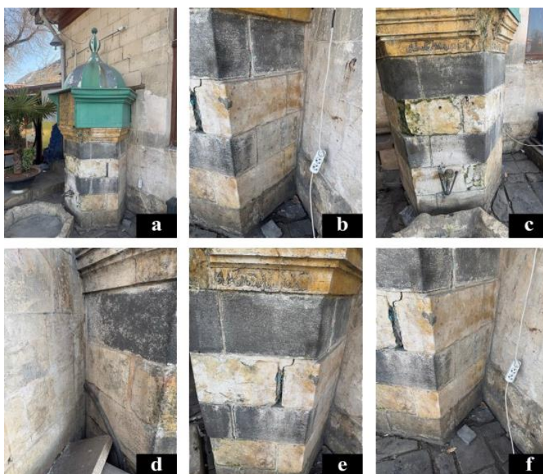
Figure 8. Chemical deterioration observed at Kumandan Fountain
