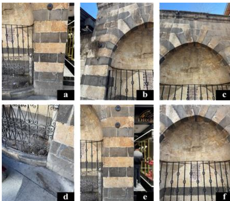
Figure 5. Physical deterioration observed at the Köseç Ahmet Ağa Fountain
