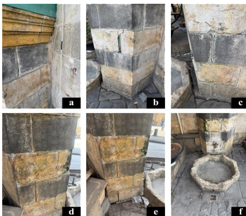
Figure 6. Physical deterioration observed at Kumandan Fountain
