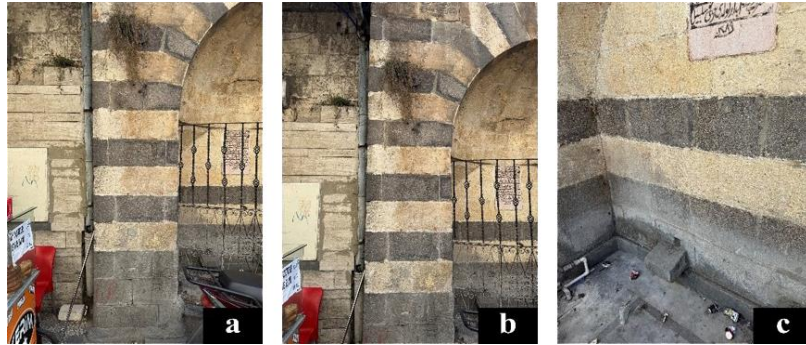
Figure 9. Chemical deterioration observed at the Köseç Ahmet Ağa Fountain.
