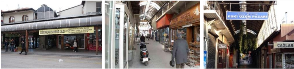
Figure 7. Top cover before the rehabilitation work
