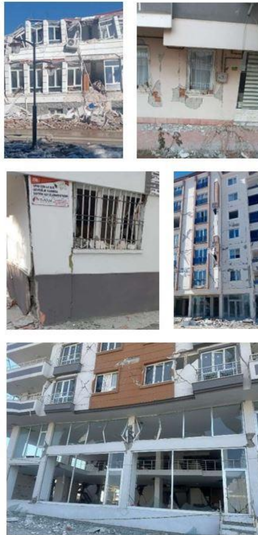
Figure 10: Short column effect
