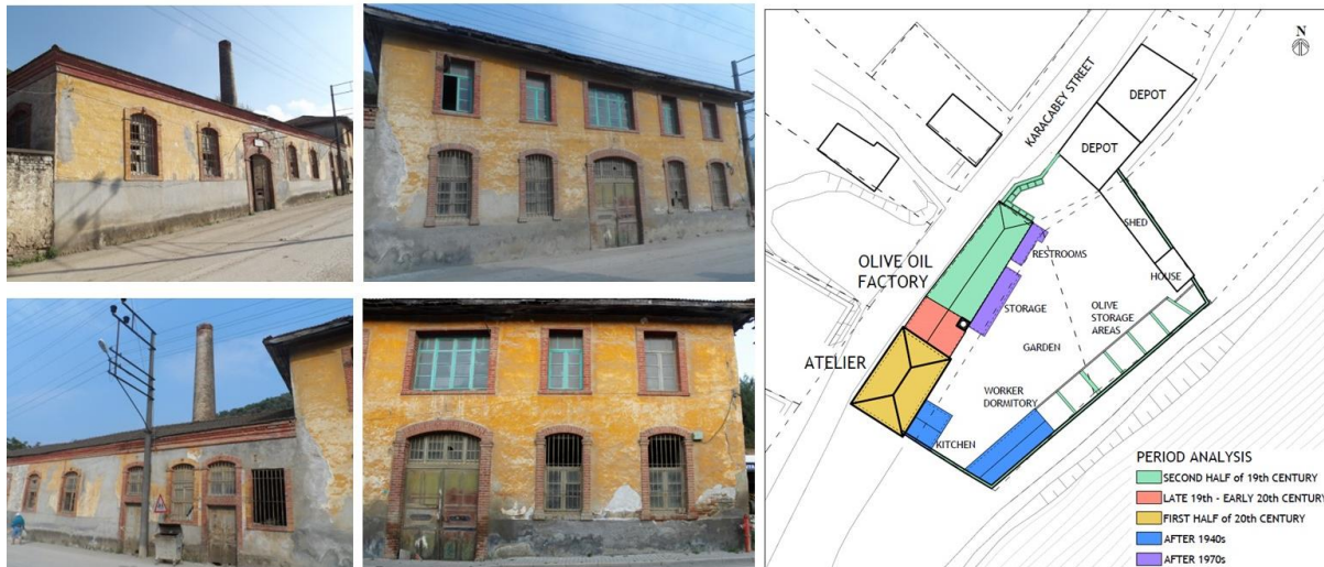
Figure 2. Photographs and site plan of Tirilye Olive Oil Factory showing the present functions of the buildings and the development of the complex in the historical process (Reproduced from Acar Bilgin, 2018)
