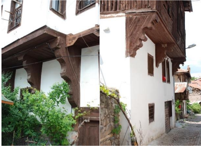
Figure 26. Examples of bracket-supported projections
