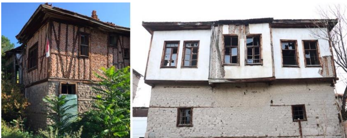
Figure 18. Examples of timber framed systems with brick and adobe infill
