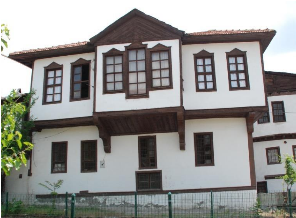
Figure 23. Guillotine and casement windows
