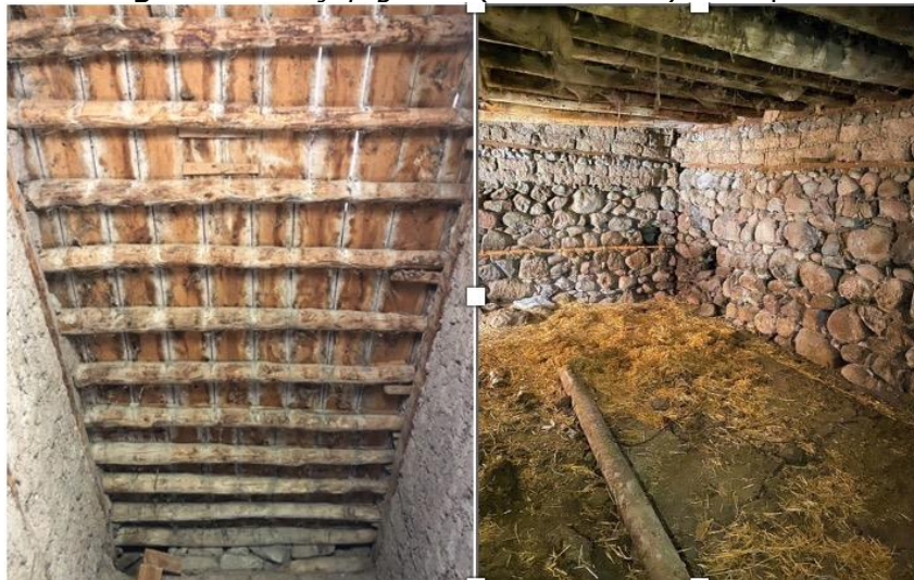
Figure 13. The ceiling of the ground and mezzanine floor
