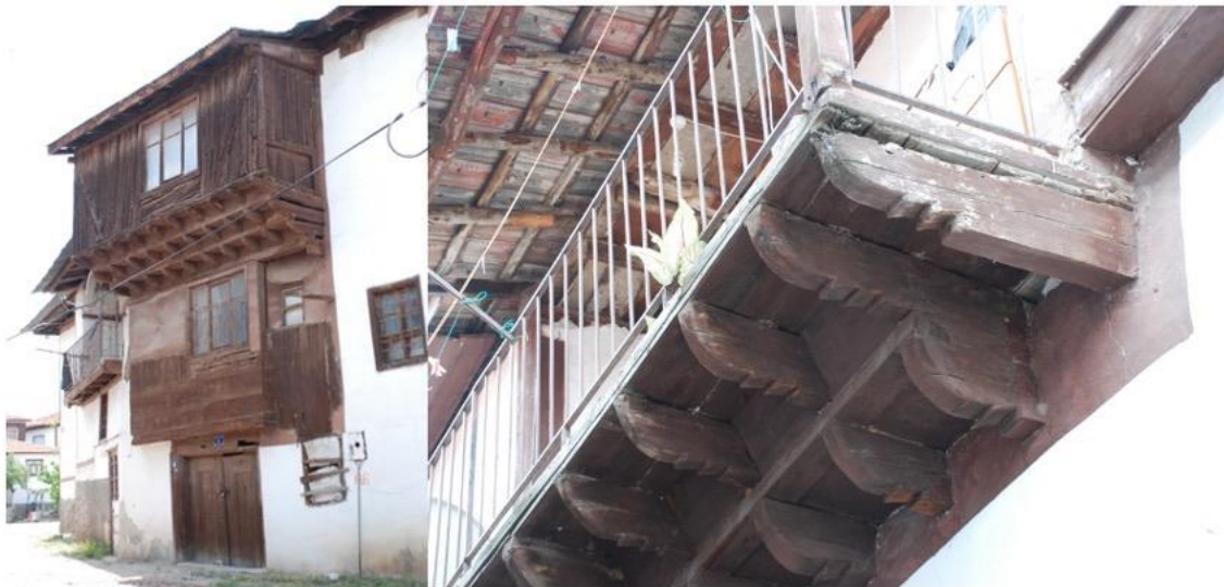
Figure 27. Examples of corbelled projections
