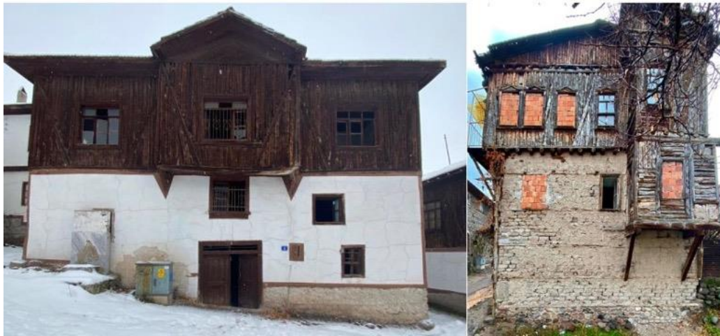
Figure 17. Examples of timber-framed systems with wood infill
