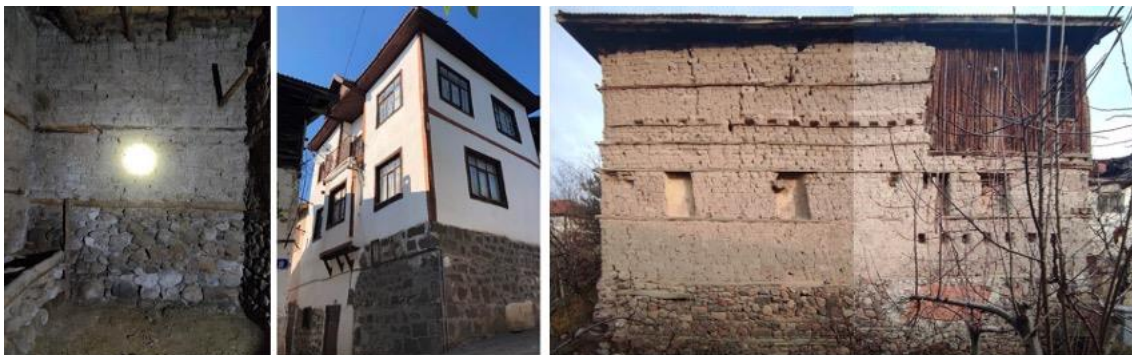
Figure 15. Examples of masonry stone walls
