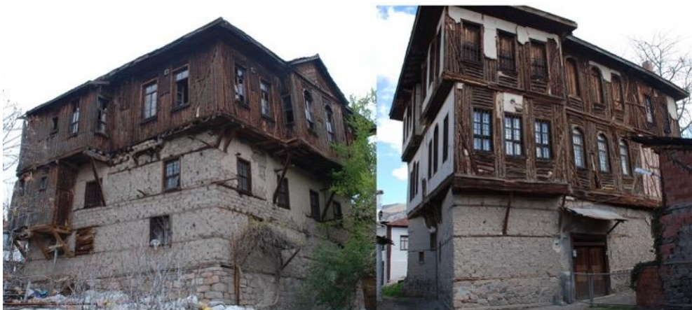
Figure 16. Examples of masonry mud brick walls
