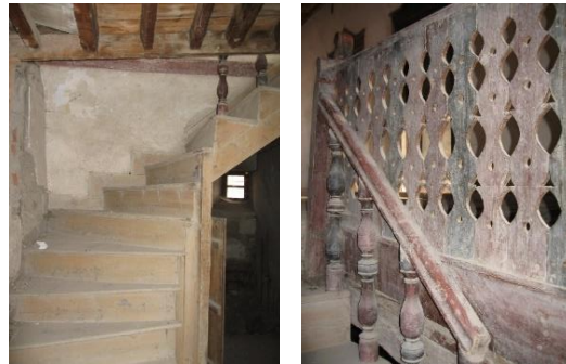
Figure 21. Example of timber staircase and balustrade.
