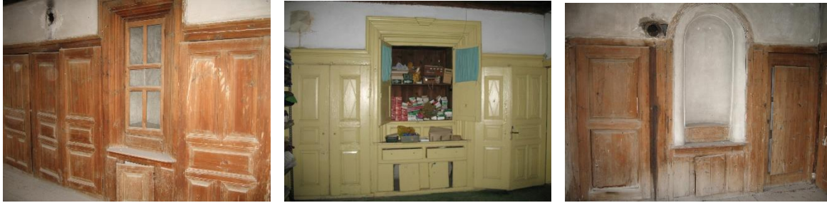
Figure 27. Examples of musandra (large cupboards for storing bedding and often built into a wall).
