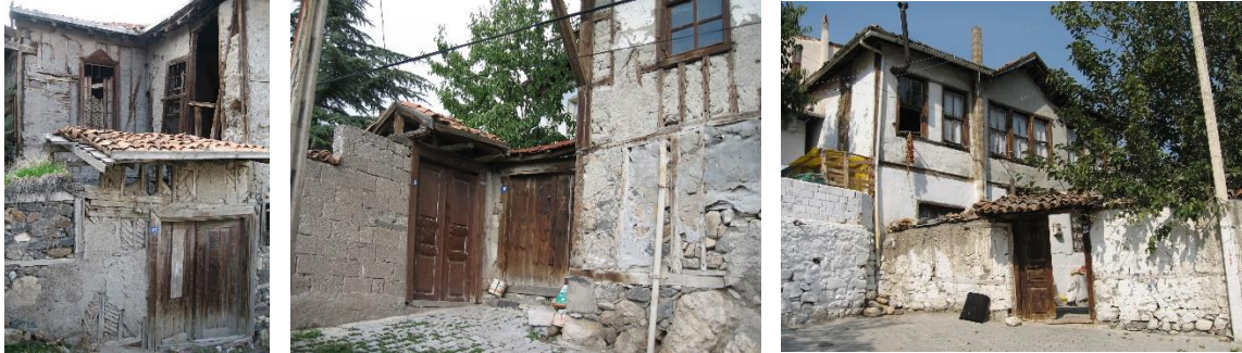
Figure 24. Examples of main doors and roofs.
