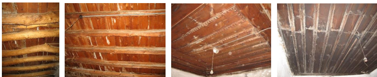
Figure 20. Examples of ceilings of depots and rooms.
