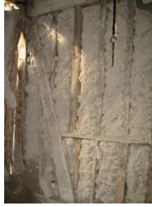
Figure 15. Timber frame construction with mudbrick infill.
