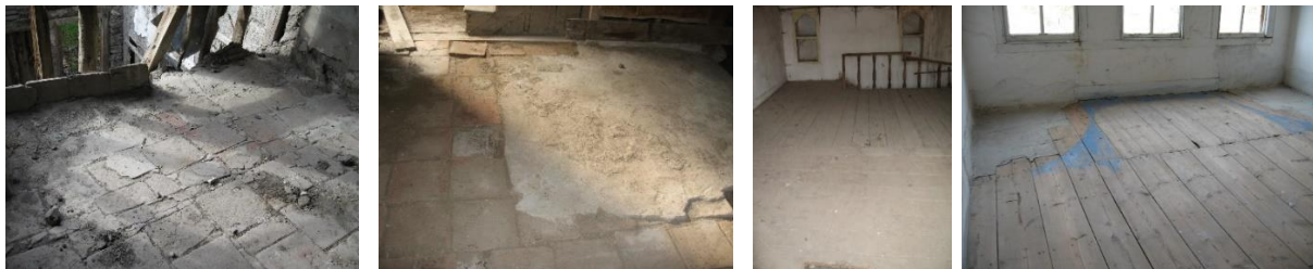
Figure 19. Examples of original terracotta tiles and timber ceiling coverings.
