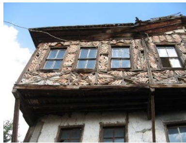
Figure 14. Timber frame construction with brick infill.
