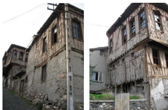
Figure 13. Examples of the "half-timber wall" ( hımış ) technique.
