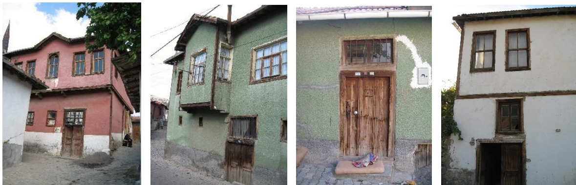
Figure 25. Examples of entrance door and top windows.
